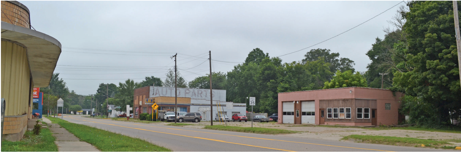
Above: The M-43 (W. Monroe Street) corridor, with the vacant structure at 600 W. Monroe shown right; Bangor, MI, 2018.
